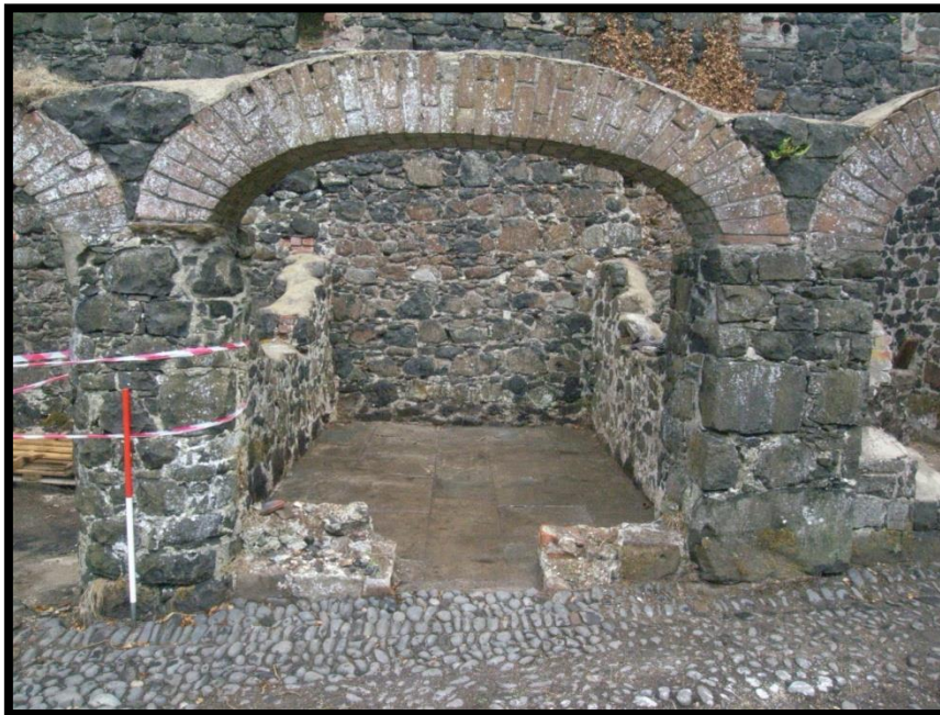
Figure 35: Bay 3 with a well-preserved area of cobbling adjacent to the entrance
