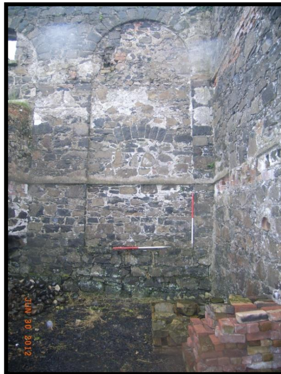
Figure 23: Circular vent and evidence for original arches
