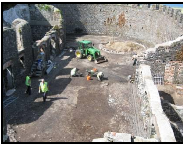
Figure 5: Gas holder uncovered within the West Yard, National Trust
