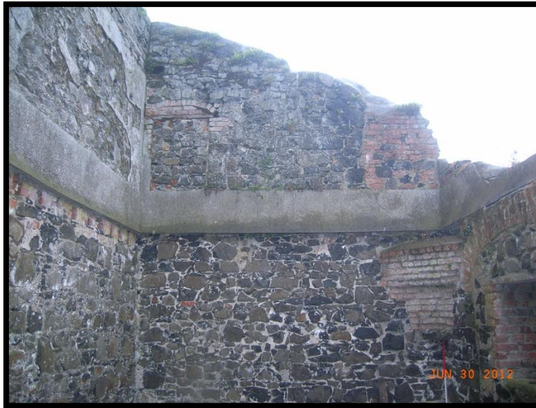
Figure 30: Concrete skirting above and red brick corbelling below
