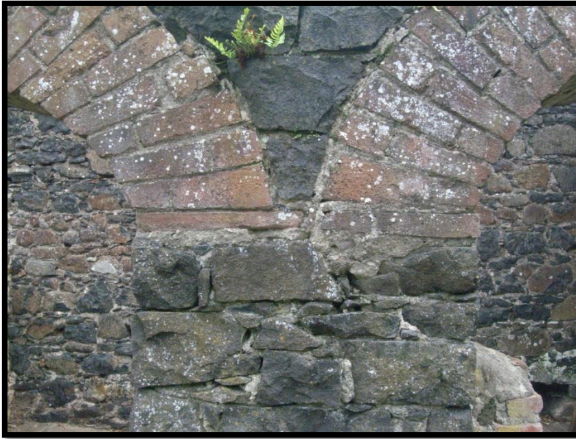
Figure 36: Well-constructed red brick arches identified in Bays 1-4
