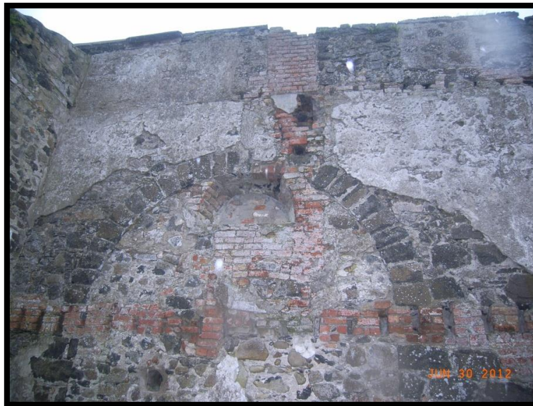
Figure 31: Original stone-edged arch within the west wall of the West Yard
