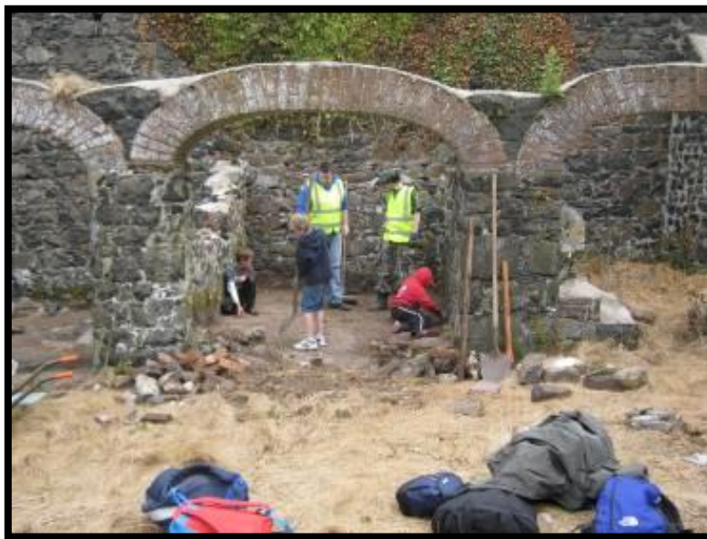
Figure 8: Arches of the West Yard during excavation, National Trust
