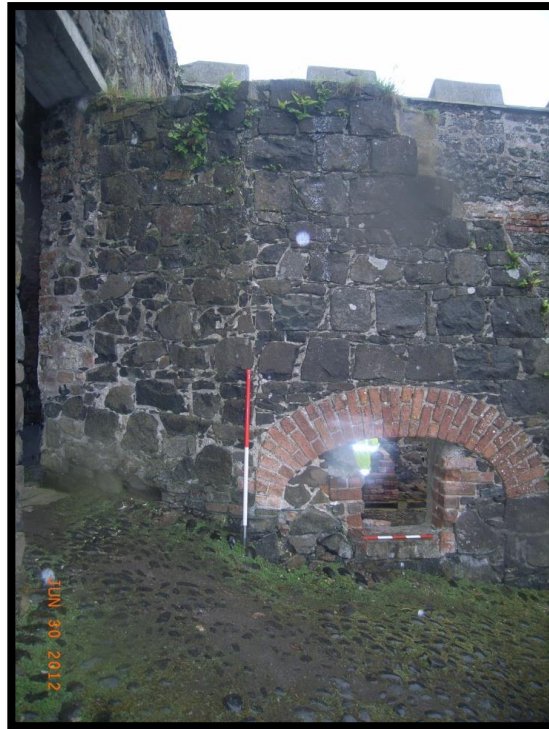
Figure 22: Doorway into stables and lower level of red brick arched window
