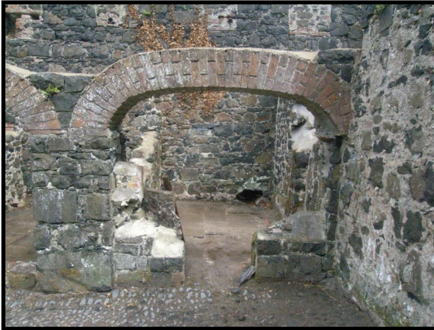
Figure 34: Bay 4 with its red brick arch, adjoined to Room 4b
