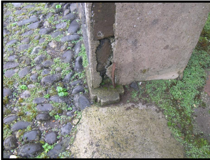
Figure 25: Decorative edging at front step of Room 2
