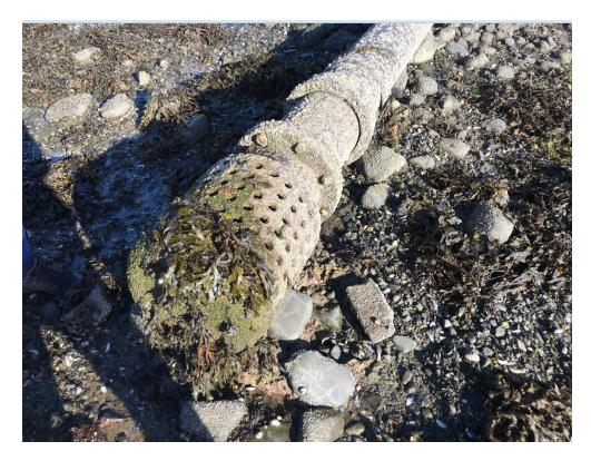
Figure 55: View of seawater intake pipe for pool, taken in October 2018. Note the supports have deteriorated and no longer support the final section of the pipe.
