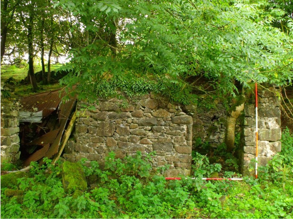
Plate 10: Possible byre at the northern end of the cottage, looking west
