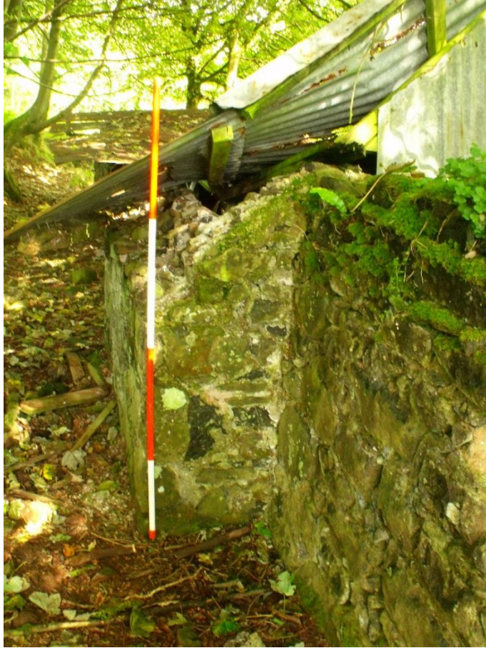
Plate 8: Bed outshot on the western side of the building, looking north
