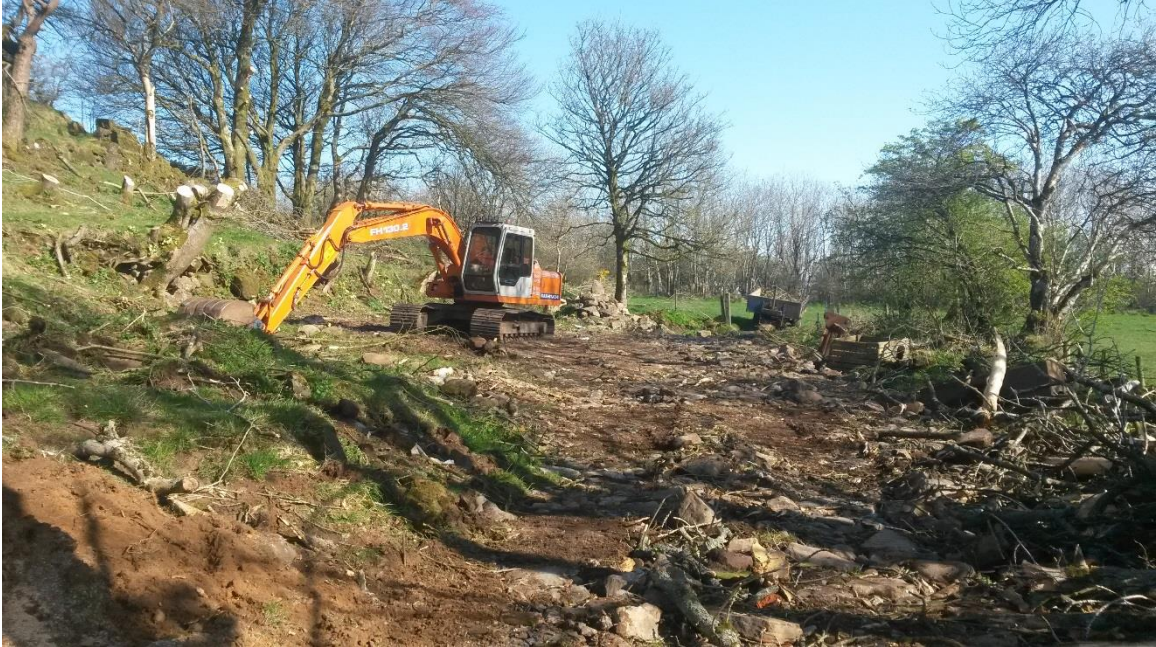
Plate 12: Monitoring work in progress, looking north
