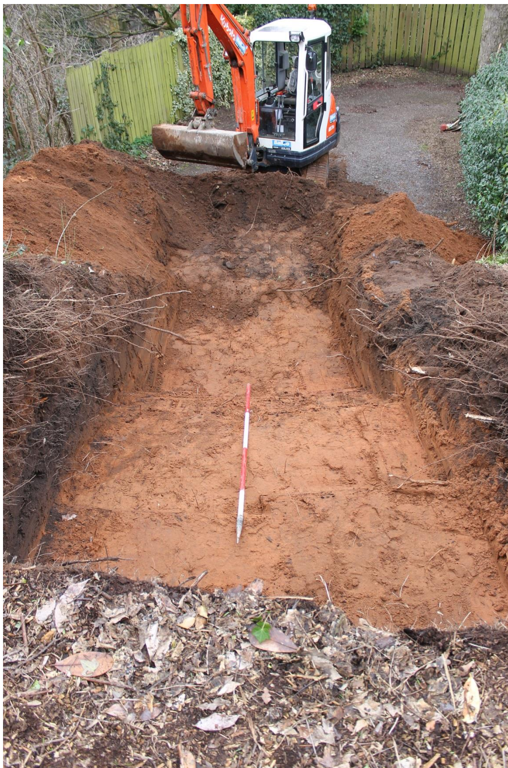
Plate 3: Trench 1, surface of the natural subsoil (c103), looking north-west
