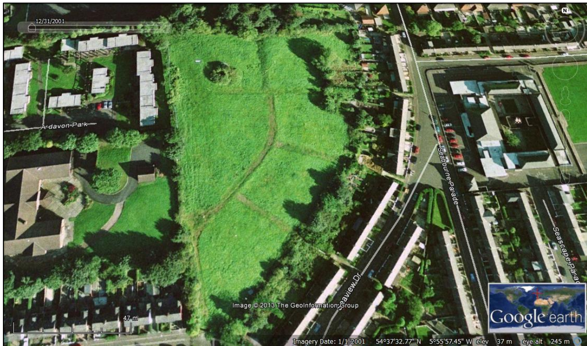
Figure 3. Aerial image of the survey area showing pathways which do not appear on any of the OS maps. Image courtesy of Google Earth and is dated 31/12/2001.
