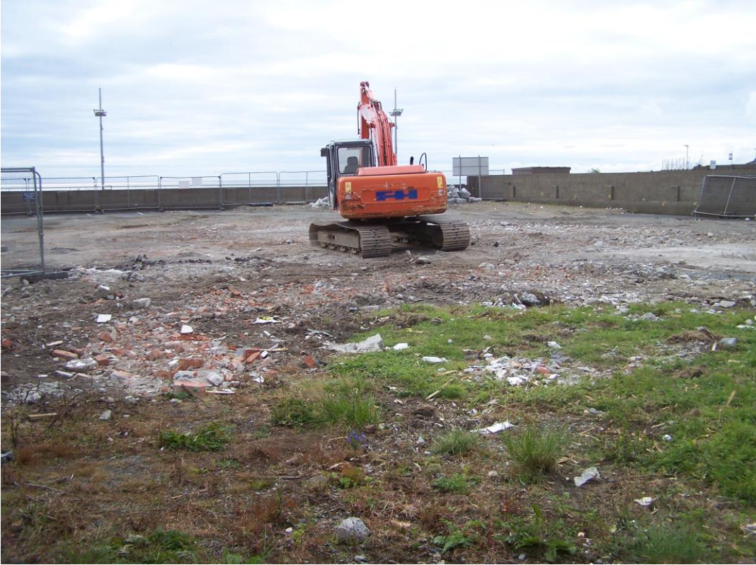
Plate 1: Site before trenches opened (looking south-east).
