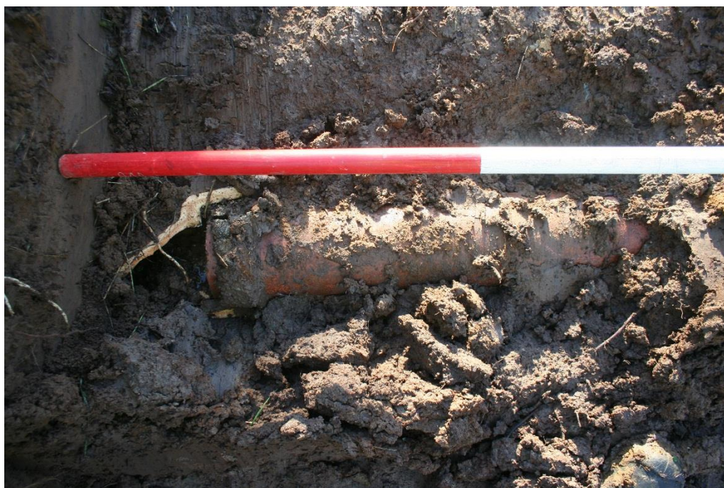
Plate 5 – The terracotta water pipe in Trench 1
