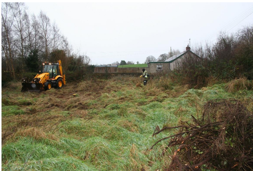
Plate 3 – General view of application site, looking south
