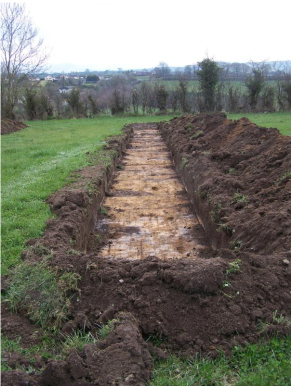
Plate 2: Trench B, post-excitation, looking south-south-east.
