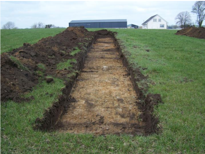
Plate 4: Trench D, post-excitation, looking north-north-west.
