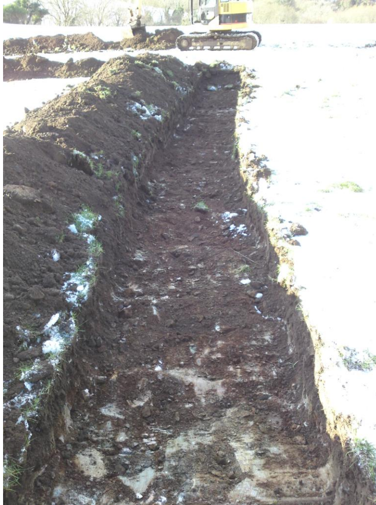
Plate 2: Trench One following excavation to the surface of the natural subsoil (Context No. 103), looking west.
