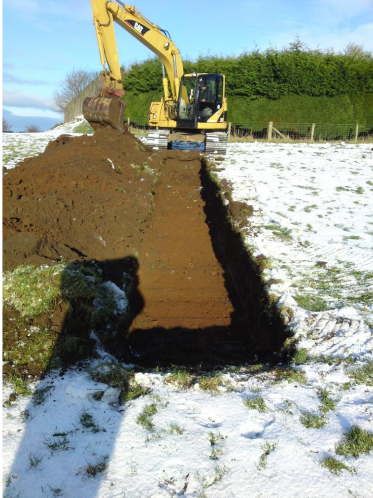
Plate 3: Trench Two following excavation to the surface of the natural subsoil (Context No. 203), looking north.
