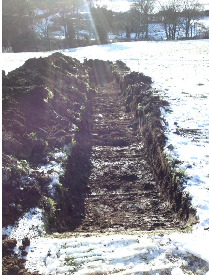
Plate 4: Trench Three following excavation to the surface of the natural subsoil (Context No. 303), looking south.
