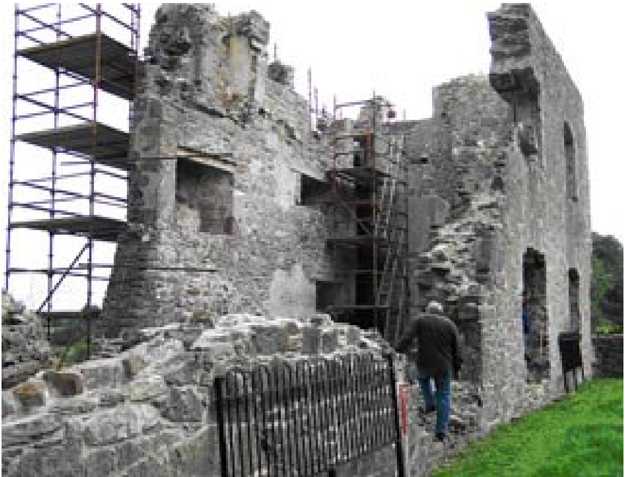
Plate Twelve: Crevinish Castle (FER 153:020), looking north-east.
