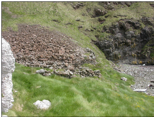
Plate 2.1: Base of slope and boat shelters looking East.
