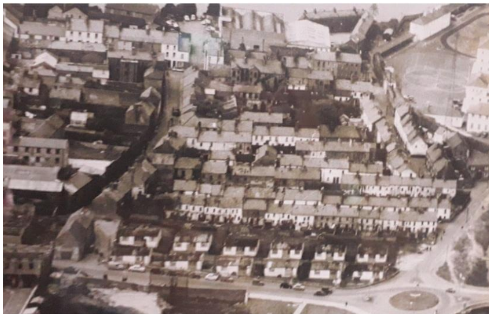
Figure 2: Mid-20 th Century aerial view of the "Backstreets" in Enniskillen
